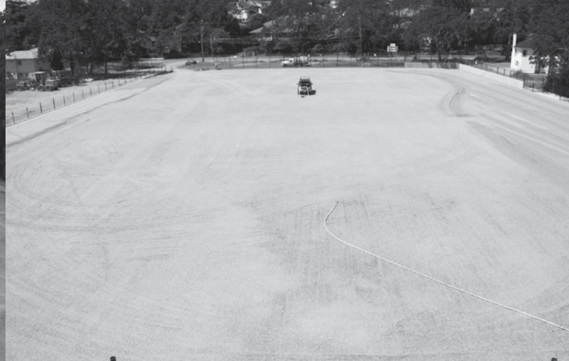
The surface ready for the turf to be installed.
