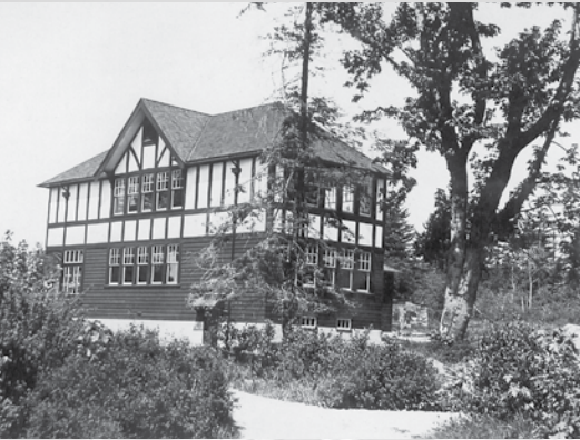
The Main classroom block was the only building on the Pemberton Woods site when it was completed in 1932.
