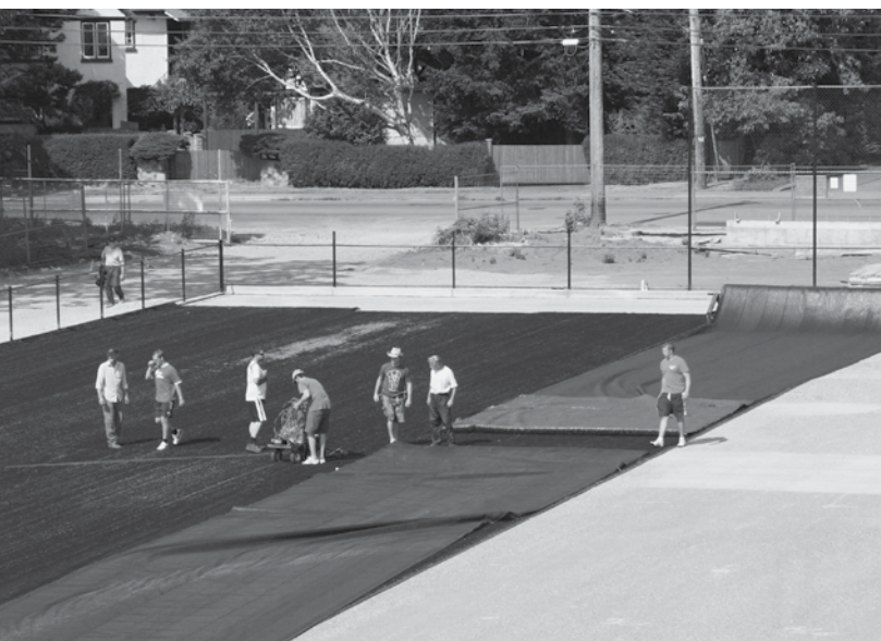
The first rolls of turf are laid.
