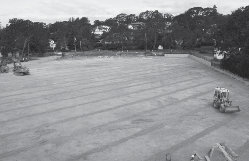
The first phase almost complete.
